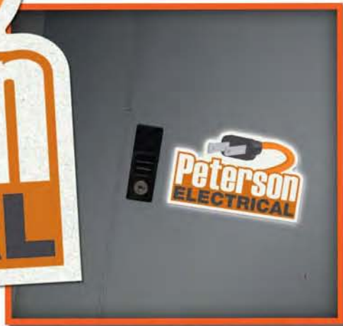
Help them find the electrical box in the dark.
